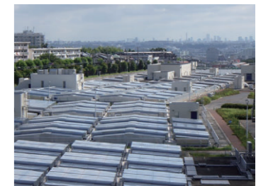
Aluminum cover installed at a water purification plant
