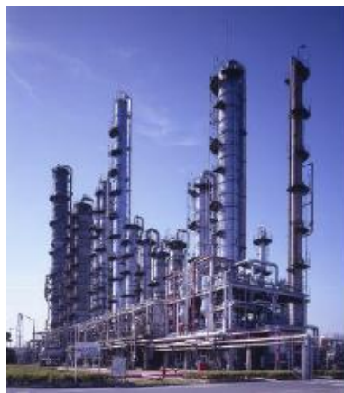
Isoprene extraction plant (Mizushima Plant)
