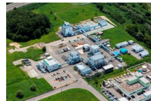
Zeon Chemicals Yonezawa Co., Ltd.
