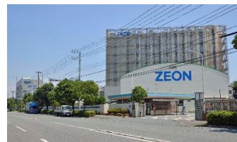
Front of the R&D Center
