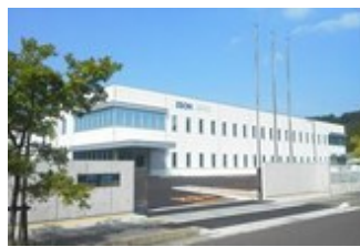
Optes Hokuriku Plant (Tsuruga Plant)
