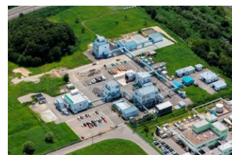
Zeon Chemicals Yonezawa Co., Ltd.
