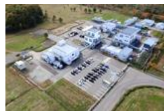
Zeon Chemicals Yonezawa Co., Ltd.
