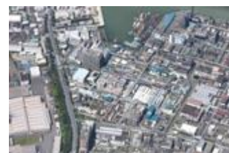
Aerial view of the Kawasaki Plant
