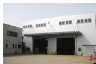
Can manufacturing and machinery plant at Zeon North Yonejima Office
