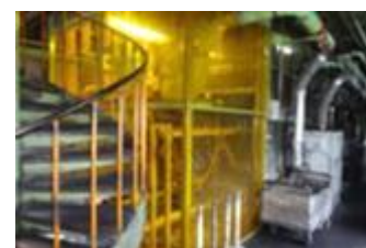
Dust containment sheet
