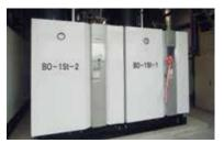
High-efficiency compact reflux boiler
