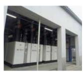
Tokuyama Plant (2014) Renewal of boiler turbine in-house power generation equipment The plant renewed all of its in-house power generation equipment to improve heat recovery efficiency and power generation output. By replacing crude oil with city gas for a portion of its fuel, the plant also reduced CO<sub>2</sub> emissions.
