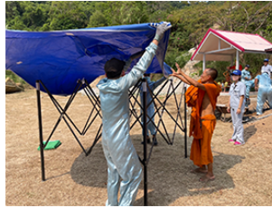
Repair work at a local temple nearby
