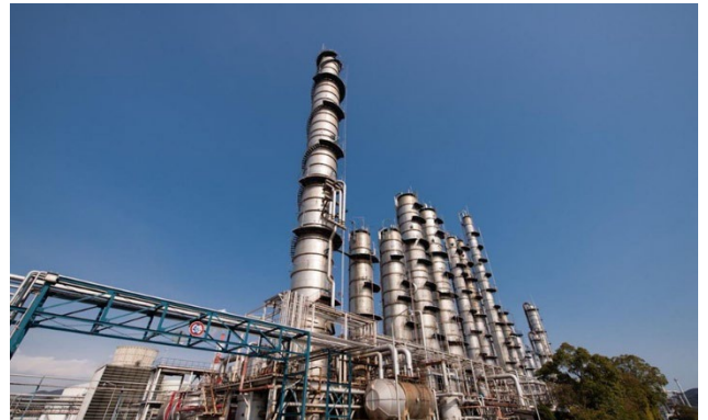
GPI plant at the Mizushima Plant
