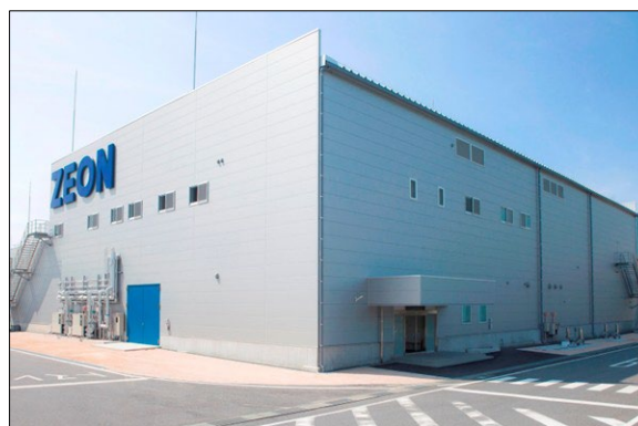
SWCNT production facility at the Tokuyama Plant
