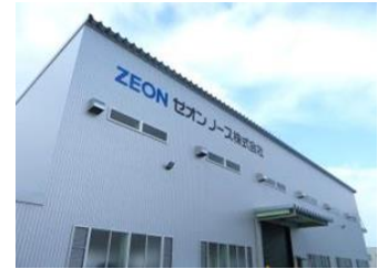
Zeon North Plant No. 5 (Completed Jan. 2016)
