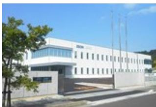
Hokuriku Plant (Tsuruga Plant)
