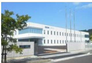
Hokuriku Plant (Tsuruga Plant)
