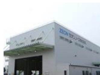
New plant (No. 4 Plant) at the Zeon North Yonejima Office
