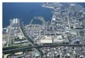
Aerial view of the Tokuyama Plant
