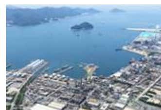
Aerial view of the Tokuyama Plant
