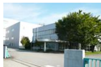
ZEON Medical's research center and plant
