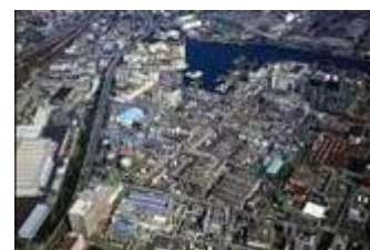
Aerial view of the Kawasaki Plant
