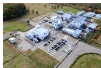
ZEON Chemicals Yonezawa Co., Ltd.
