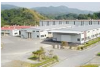
ZEON Kasei's Yamaguchi Plant
