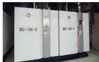
High-efficiency compact reflux boiler
