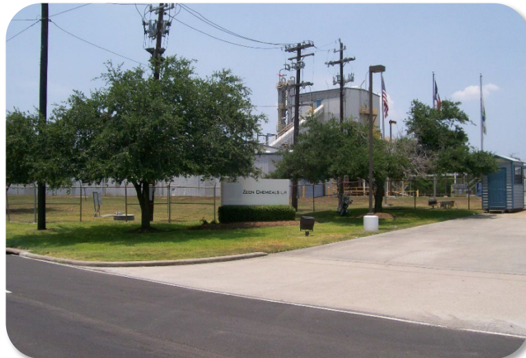
Texas Plant, Zeon Chemicals L.P.
