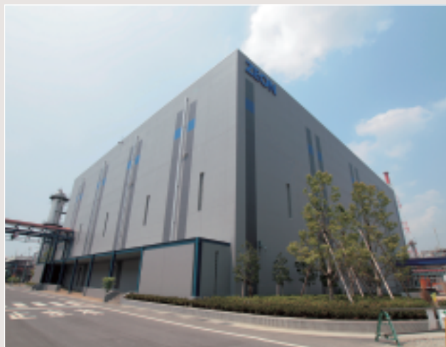
Integrated Production Center
