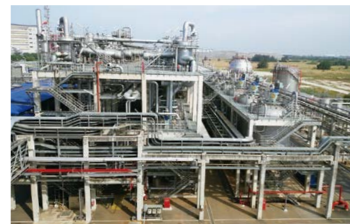
S-SBR production plant(Second Plant of Zeon Chemicals Singapore)
