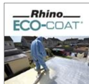
Polyurea coating for rooftops Eco-Coat
