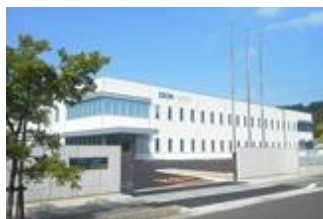
Hokuriku Plant (Tsuruga Plant)
