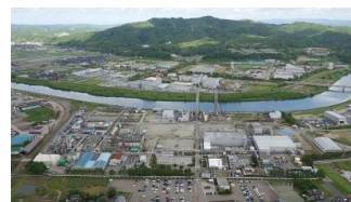
Aerial view of Takaoka Plant
