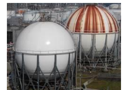
Repainted tank (foreground, Zeon Corporation's Tokuyama Plant)
