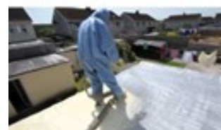
Polyurea coating for rooftops Eco-Coat
