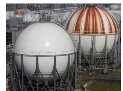
Repainted tank (foreground, Zeon Corporation's Tokuyama Plant)
