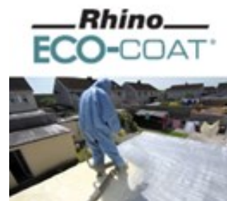
Polyurea coating for rooftops Eco-Coat
