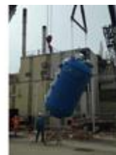
Installation of new acrylic rubber reactor in Kentucky.
