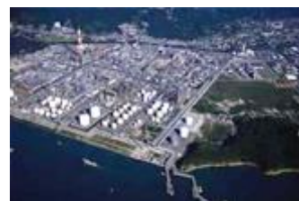
Aerial view of the Mizushima Plant
