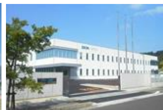
Optes Hokuriku Plant (Tsuruga manufacturing plant)
