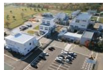
ZEON Chemicals Yonezawa Co., Ltd.
