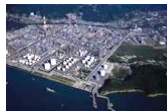
Aerial view of the Mizushima Plant
