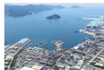
Aerial view of the Tokuyama Plant
