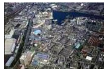
Aerial view of the Kawasaki Plant
