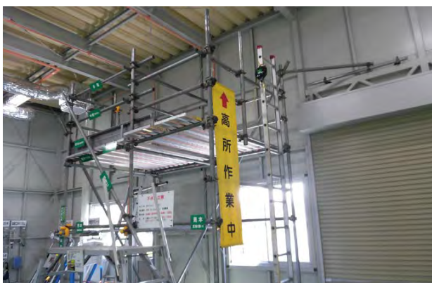
Display in the Safety Workshop showing how to use scaffolding
