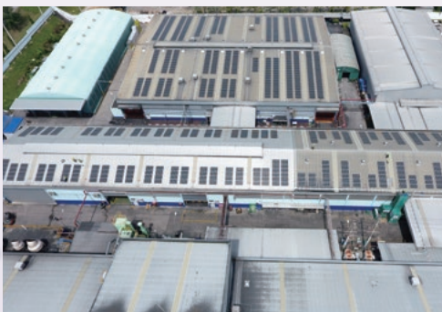
At Zeon Advanced Polymix Co., Ltd., solar power is generated on the plant's roof.
