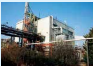
Zeon Chemicals Europe Ltd. U.K. Plant
