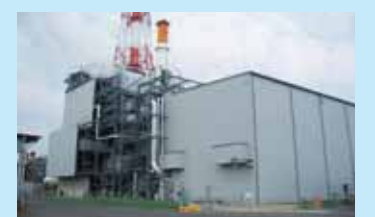
Energy conservation plan for the Mizushima industrial complex
