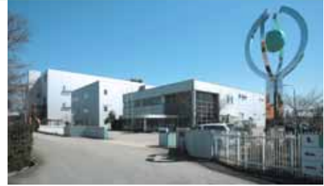
Overall View of the Plant
