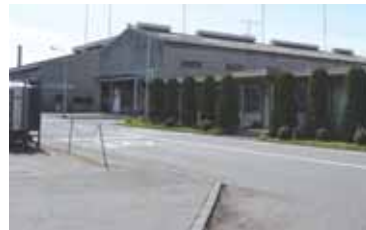
Overall View of the Offices
