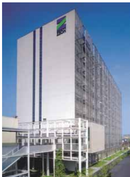
New Facility (No. 10 Building)
