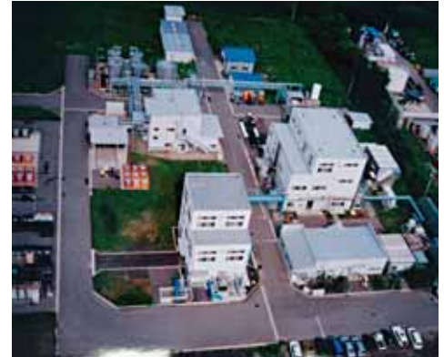
Overall View of the Offices
