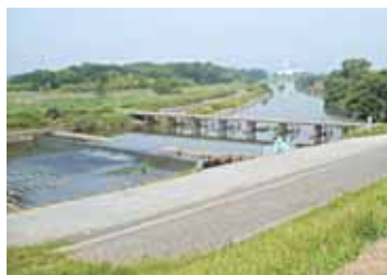
Opegawa River and wooden bridge (near Kawagoe Plant)
