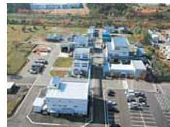
Overview of facility
