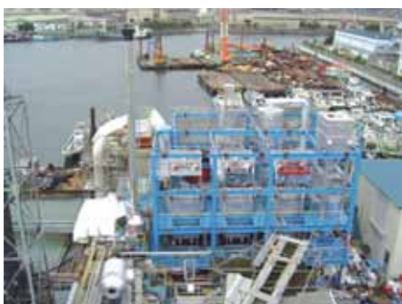
Incinerator under construction
