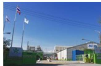
Zeon Chemicals (Thailand) Co., Ltd. (ZCT)
